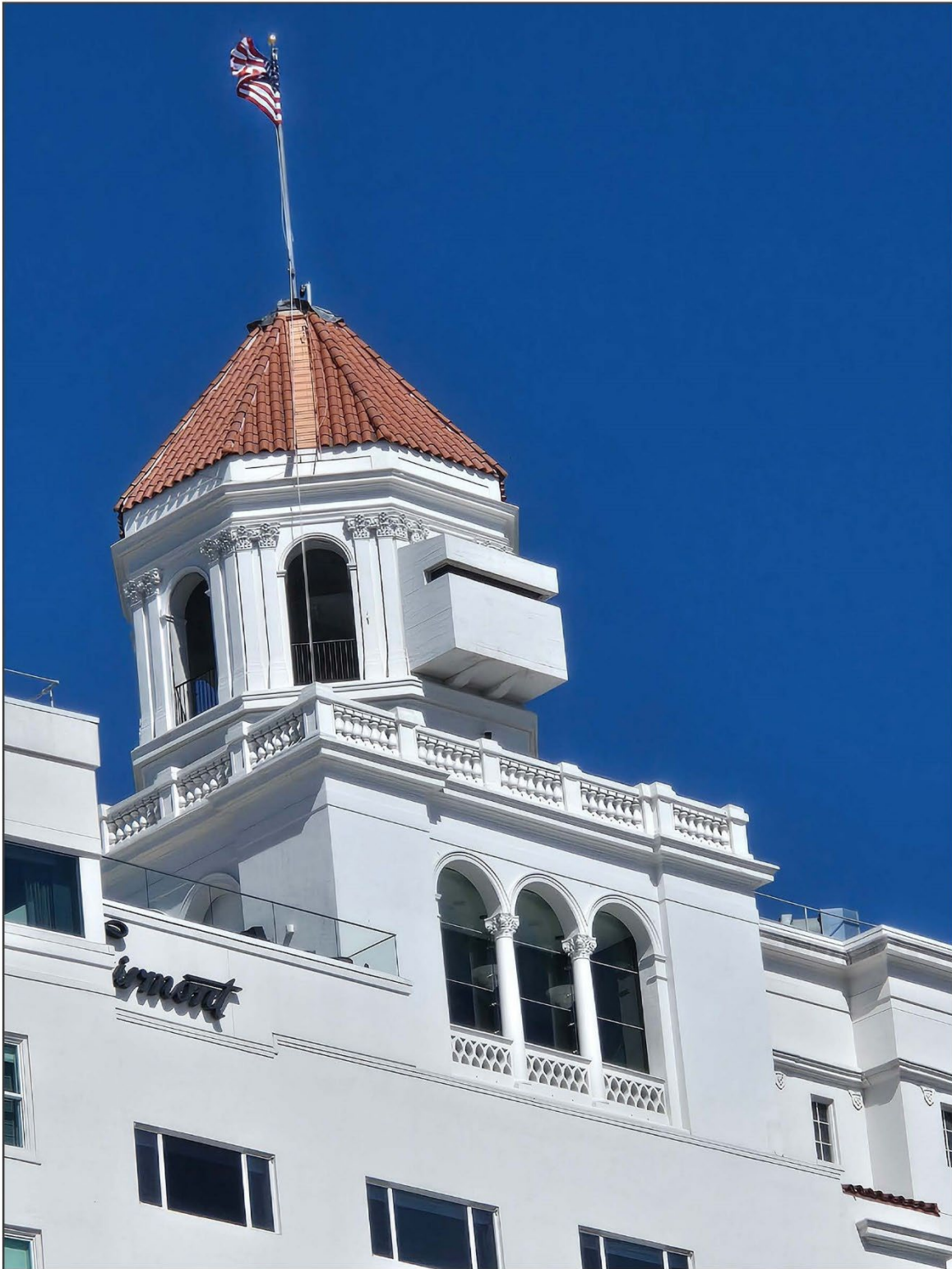
4. View northeast of pavilion, lantern, and pillbox
