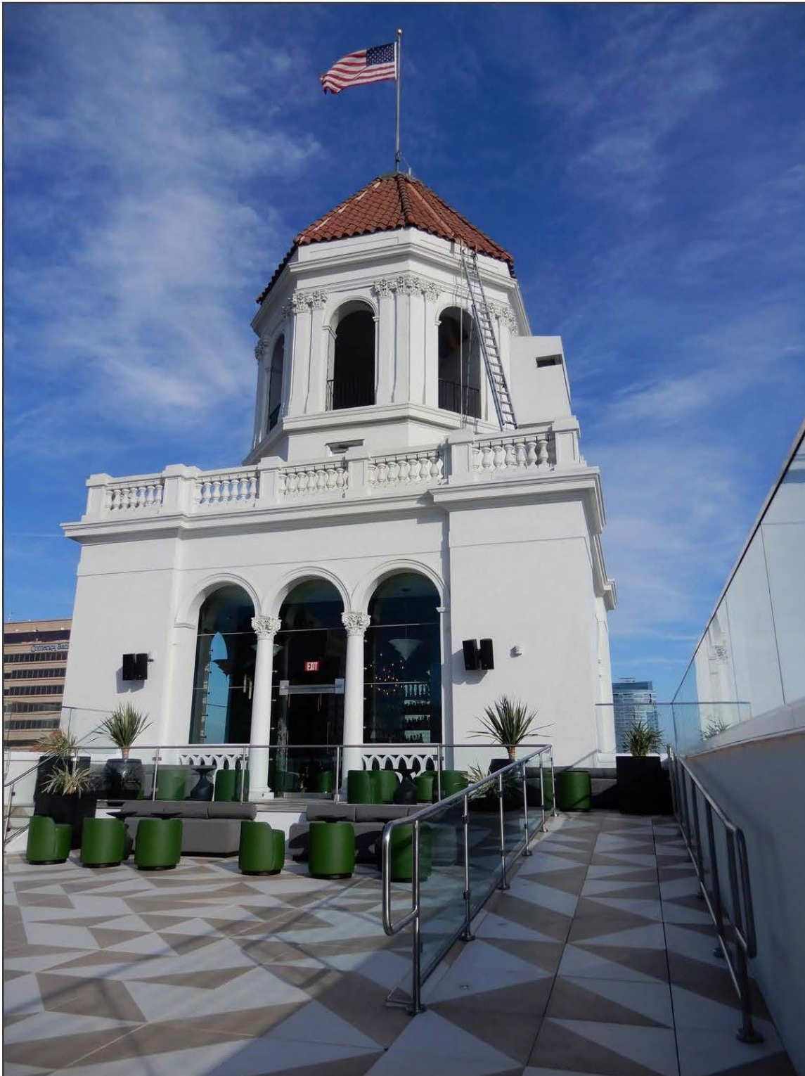
29. 14th floor, rooftop deck looking east toward pavilion
