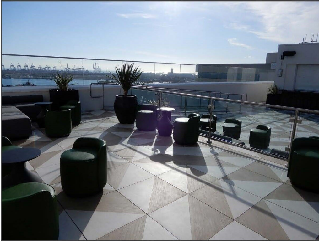
28. 14th floor, rooftop deck looking southwest
