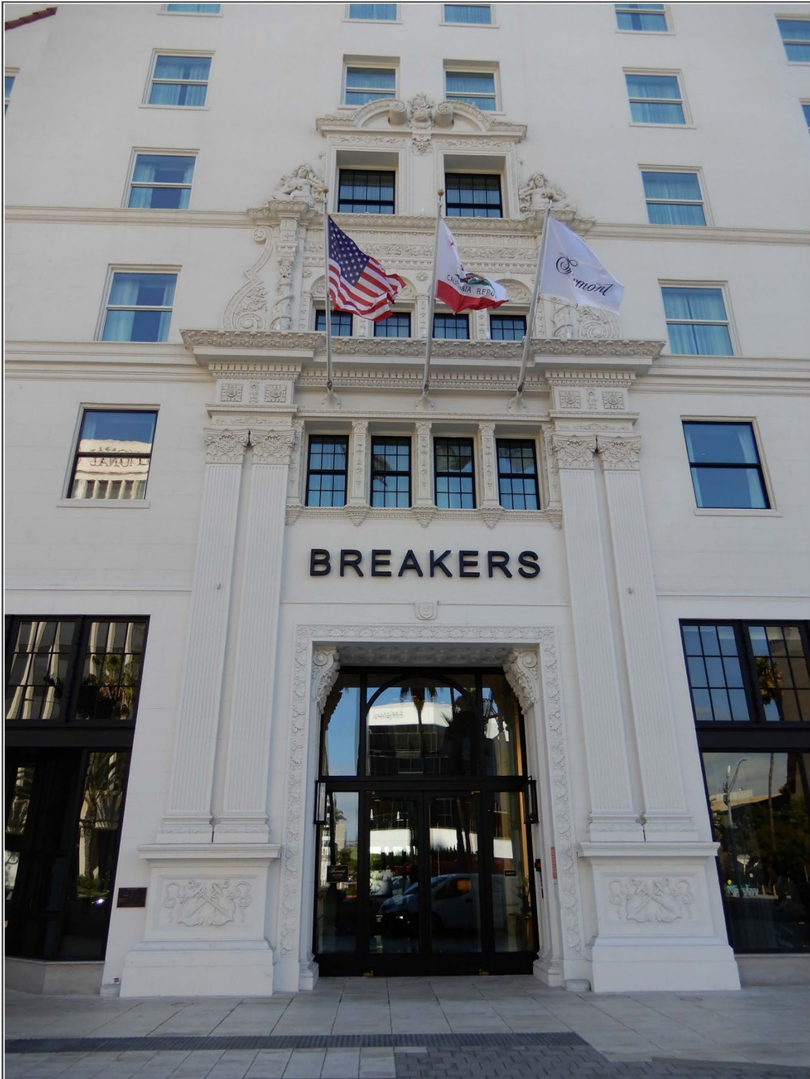
3. View south of primary (north) façade entrance portal
