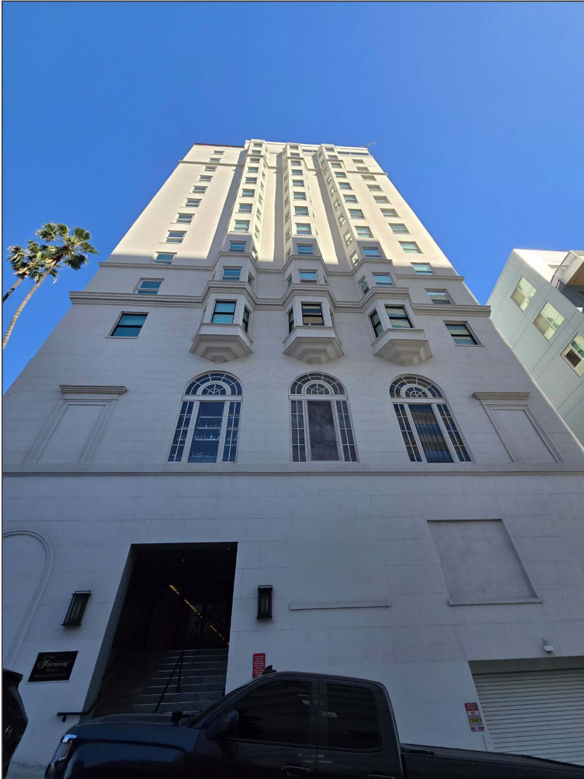
5. View east of west elevation
