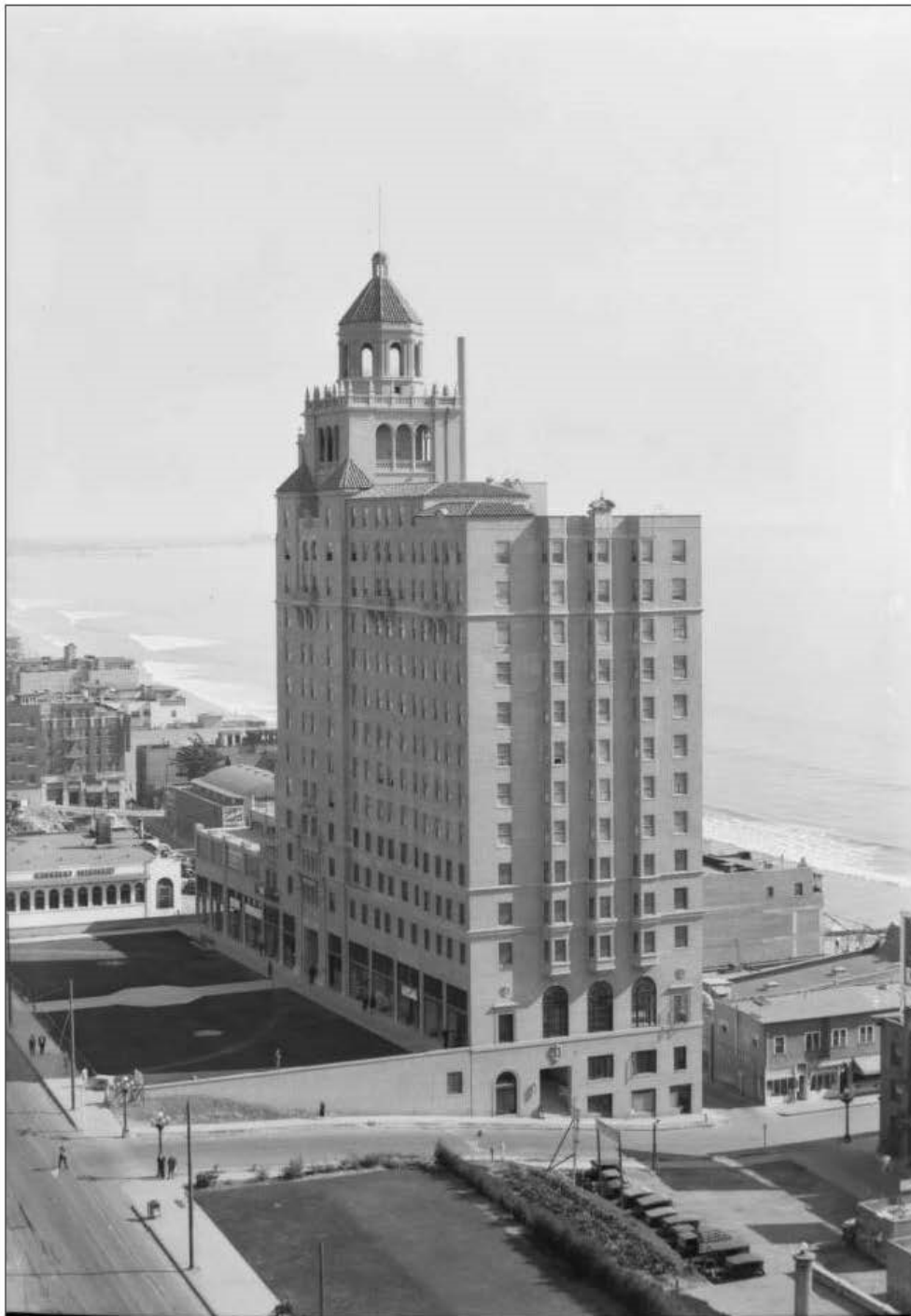
Fig 2. View from northeast, "Breakers Hotel, 210 East Ocean Boulevard, Long Beach, CA, 1926." USC Libraries.
