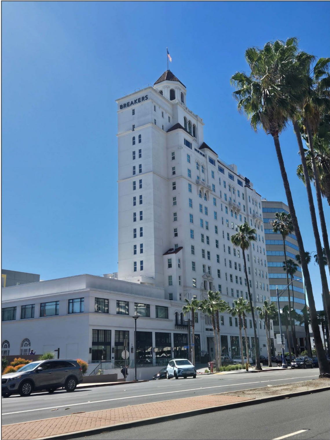
2. View southwest of primary (north) façade and east elevation from East Ocean Boulevard
