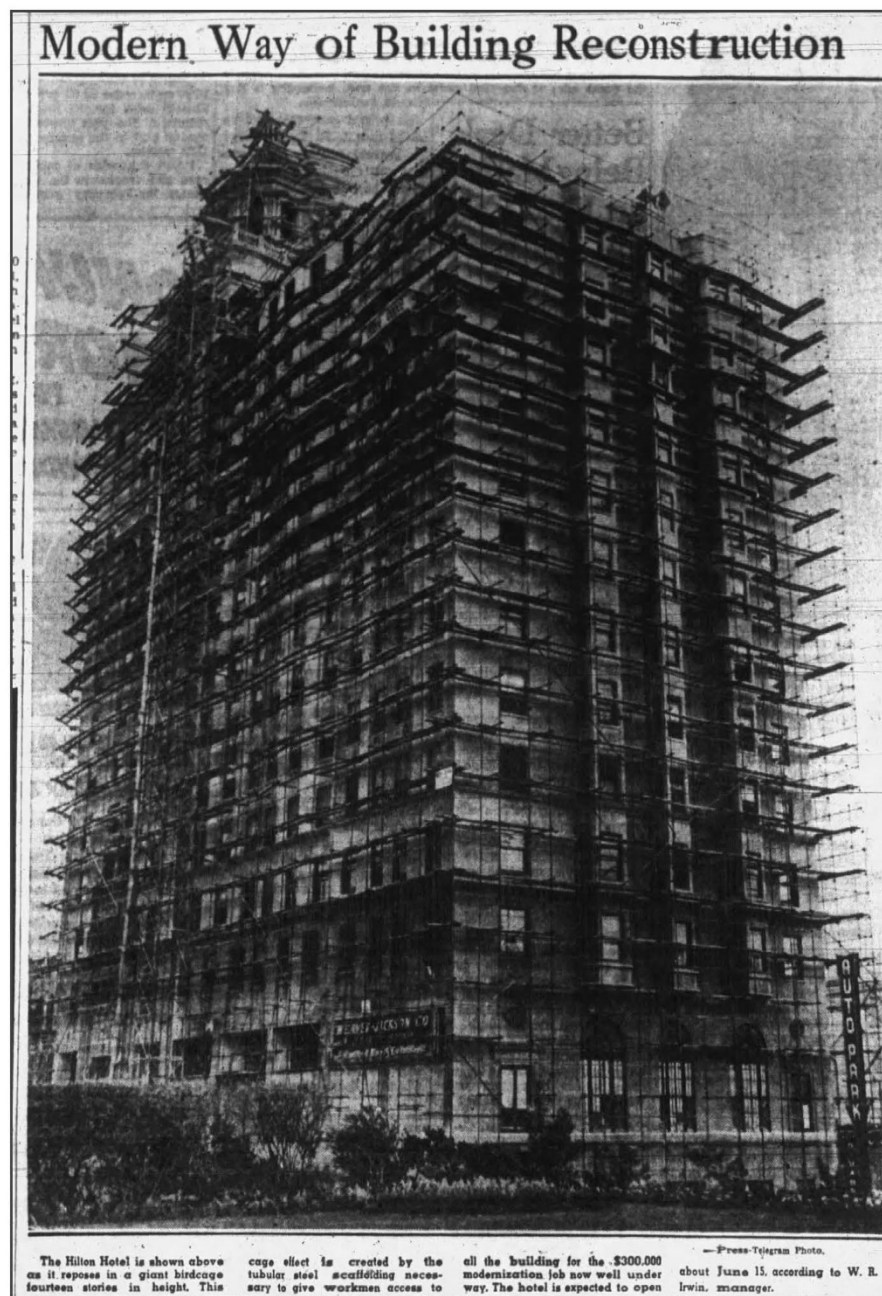
Fig 5. March 26, 1939 images of the former Breakers Hotel enveloped in scaffolding in the Long Beach Press-Telegram newspaper, accessed from newspapers.com.
