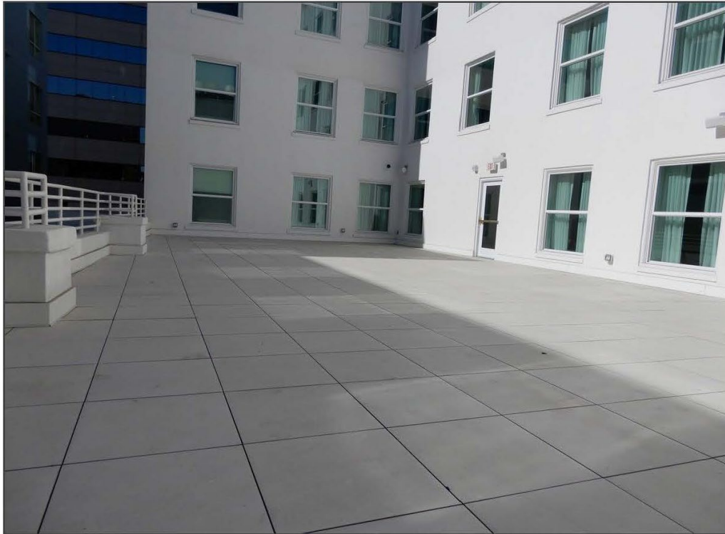
20. 2nd floor terrace, looking west
