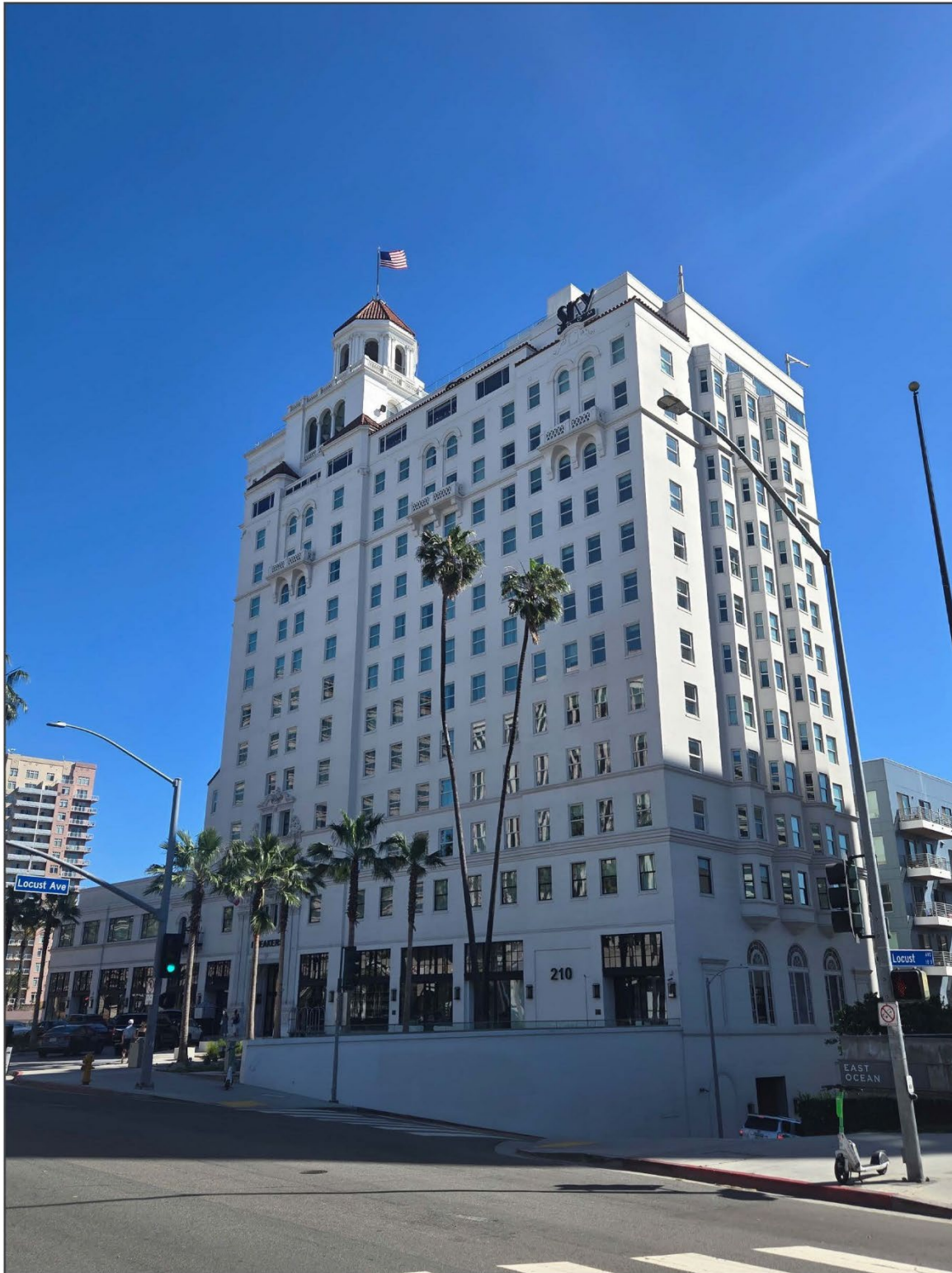
1. View southeast of primary (north) facade from East Ocean Boulevard
